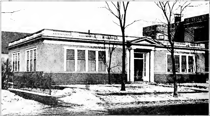
FIG. 2. EXTERIOR GRAMMAR SCHOOL BUILDING FOR MANUAL TRAINING AND DOMESTIC SCIENCE, EVANSTON, ILLINOIS.
